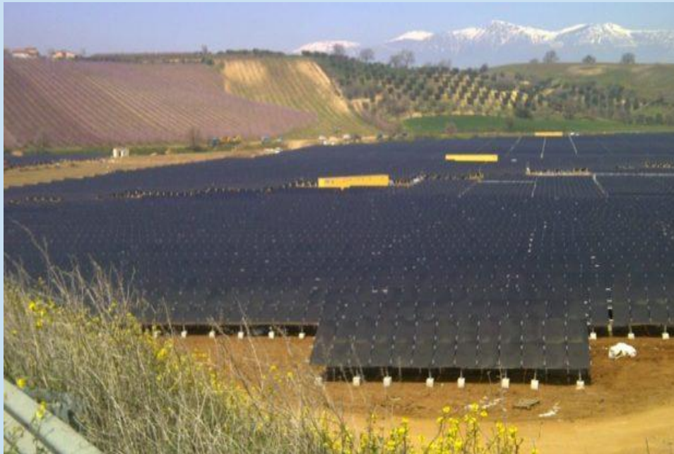
Figure 23 : PICTURE OF THE CHILEAN SOLAR PV PROJECT
